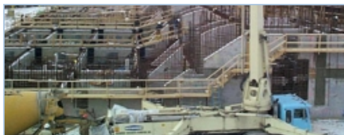
Floatable section under construction (Feb. 2001)
