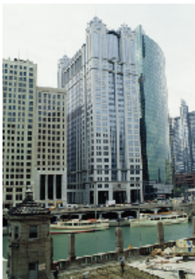
With column mixes carrying design strengths in excess of 10,000 psi, Chicago's 225 West Wacker Drive was among a wave of late 1980s-early 1990s buildings to incorporate high-strength concrete.
